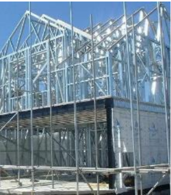
Cladding & light steel framing
